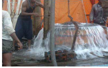
Artesian well in volcanic aquifer near Addis Q = 115 l/s
